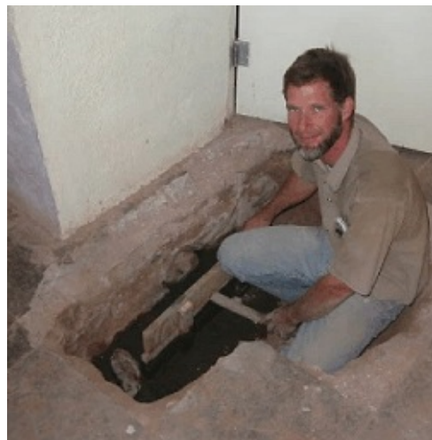
Floor/foundation work (David)
