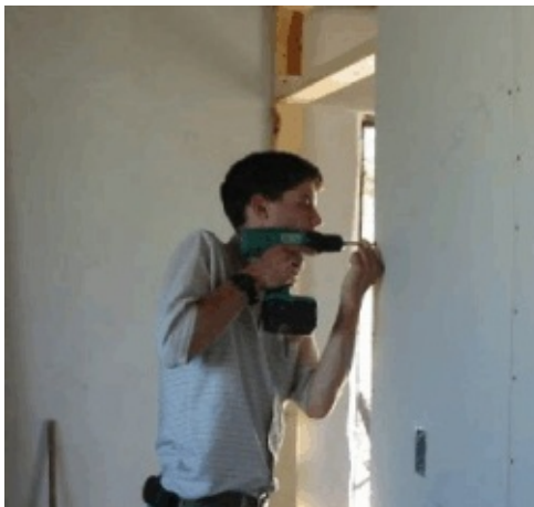
Phil putting up drywall at David's
